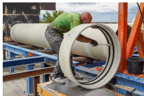
Fig. 25 b) Reka coupling in preparation for installation on an end of a GRP pipe
