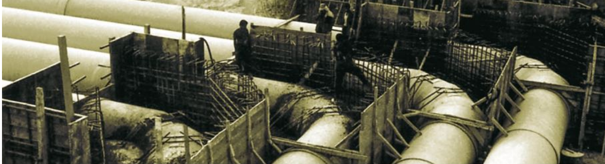
Fig. 41 Joined pipes with angular deflection
