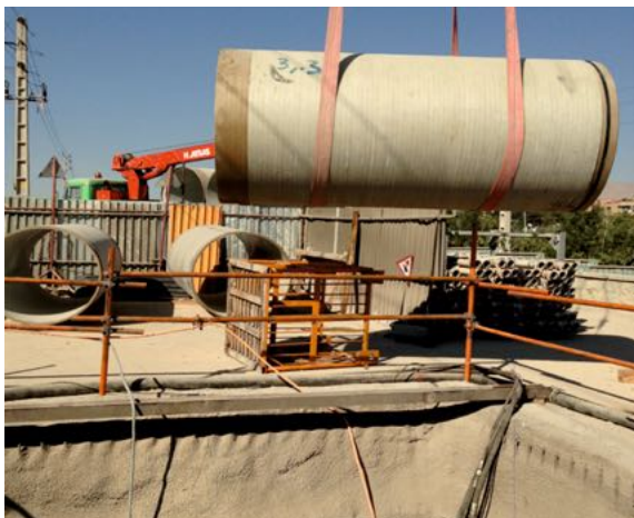
Fig. 19 Jacking pipe ready for installation
