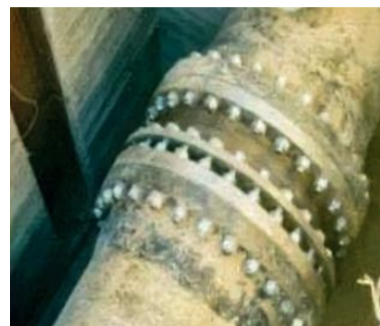
Fig. 30 b) Flanges installed on pipes
