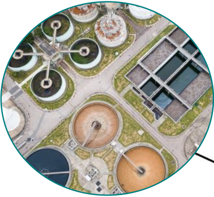
potable water treatment plants
