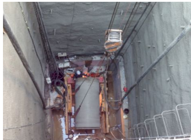
Fig. 20 Jacking pipe lowered in the working base
