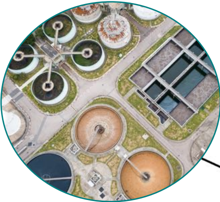
potable water treatment plants
