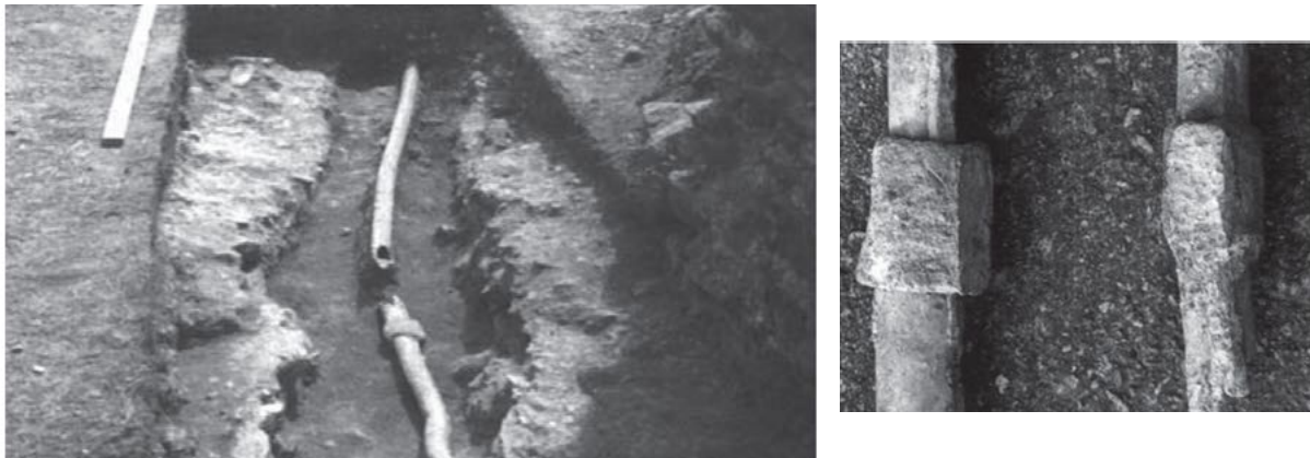
Fig. 2 a) Lead Pipes, b) Separately cast fittings - Sarmizegetusa (photo Piso, G. Băeșan 2000)
