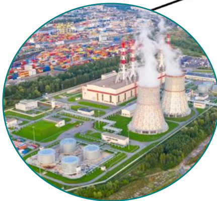
steam power plants
